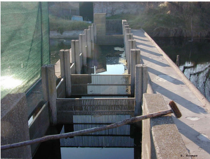
Pumping locations in source water waterways should be separated from pond effluent sites and have limited exposure to animal wastes. Filtering the water is essential to reduce predators.
